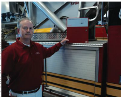
ILSS President Brian Sheely poses at a local fire department with Honeywell's IPGSM-DP fire alarm communicator.
